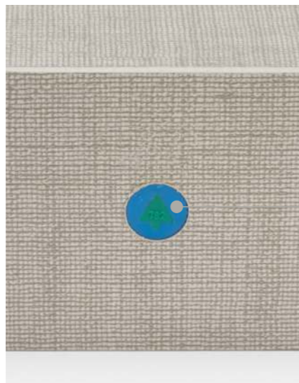
Typical Q-Mark 3rd party fire door identification
